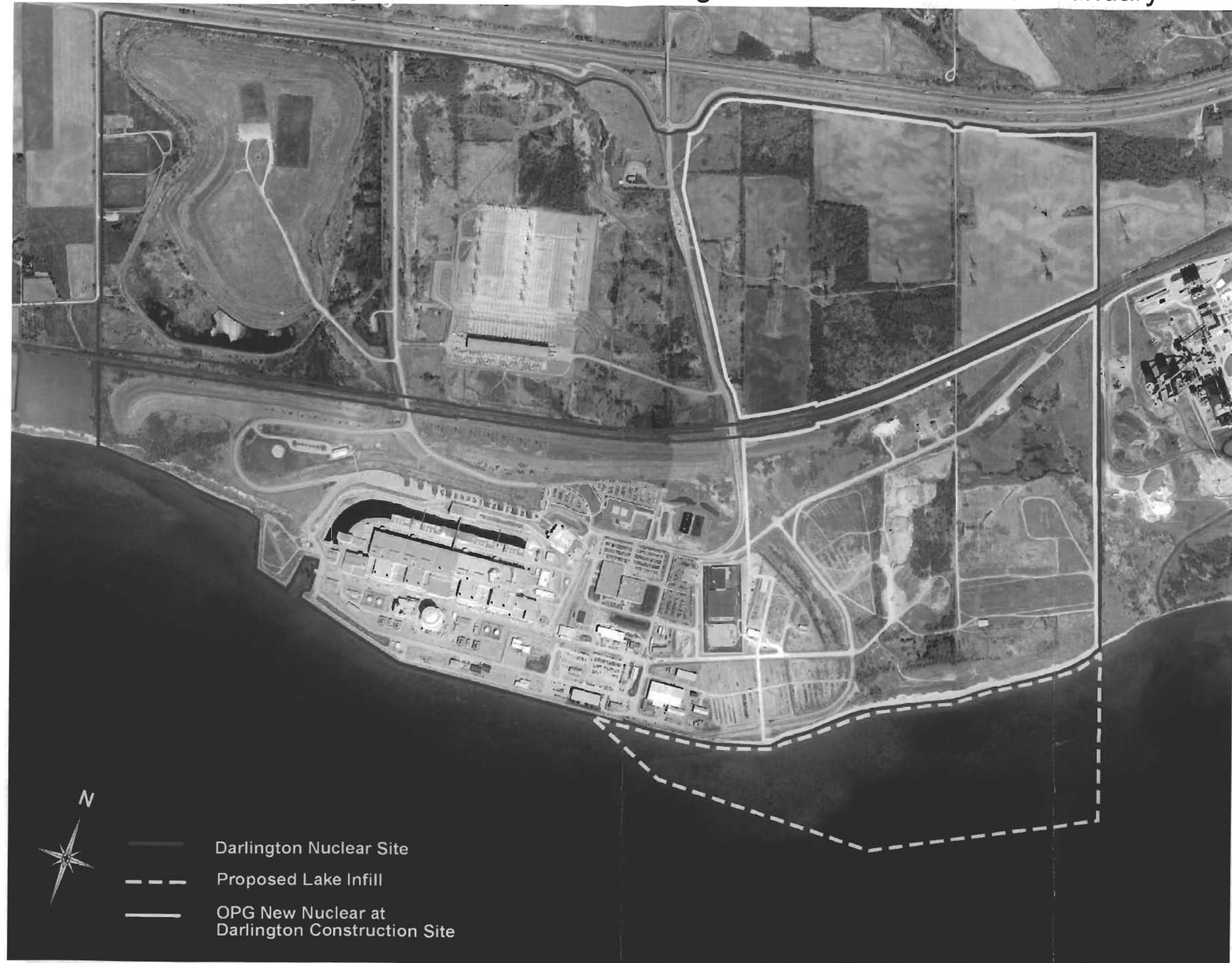
Figure 1.4-3 Photograph of DN Site Illustrating NND Construction Site Boundary
